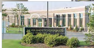
Canada, Toronto Plant-1
